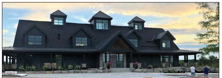
The clubhouse as seen from the main entrance.
