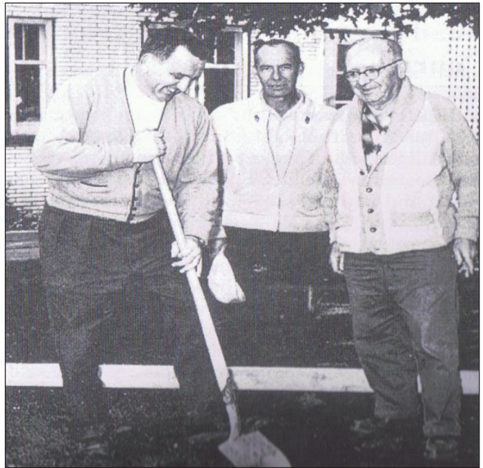
Building committee chairman Hank Smith officially turned the sod for the new Saugeen clubhouse in September of 1965. Also in the photo are contractor Burt Urquhart and club president Arthur Maundrell. The facility served the club well for many years but with a growing membership an upgrade and expansion was needed. The club spent $1.85 million on the project and the renovated clubhouse opened in June 2013.
